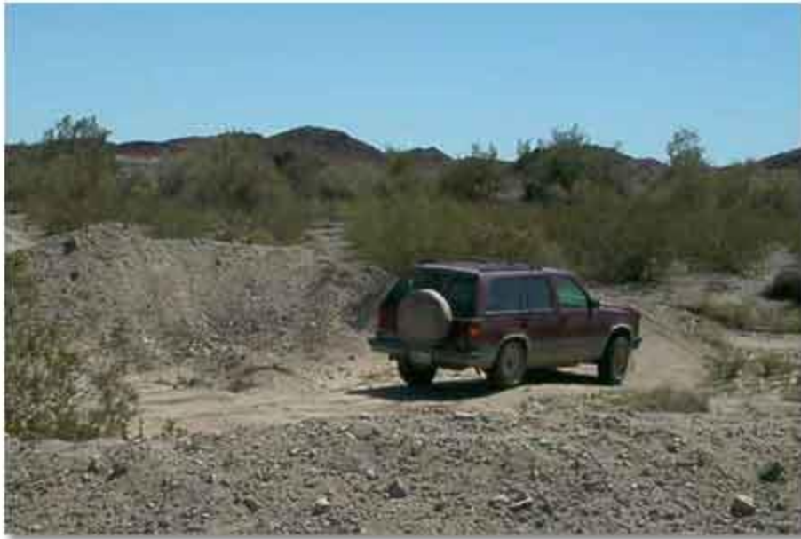
Piles of earth blocking the road to the Black Agate Thunderegg Mine.
